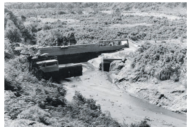
The original dam in 1917.
